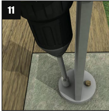
11 Attach the aluminium foot plate to the concrete pad foundation and fix using an appropriate anchor fixing - ensure plate lines up with the oak post.
